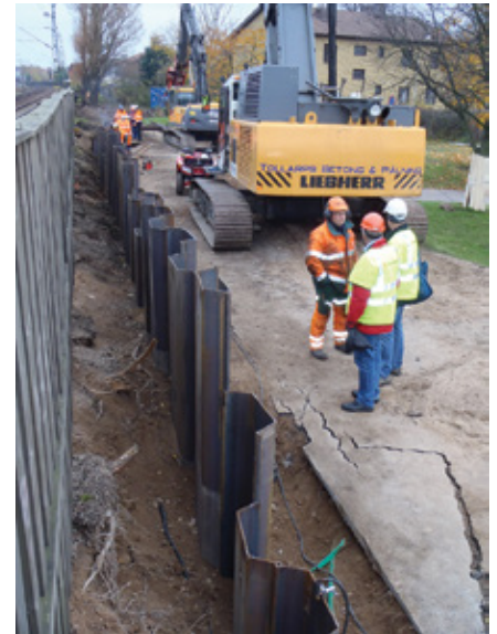
Figure 2: Installation of the sheet pile wall in Furet (Sweden)
