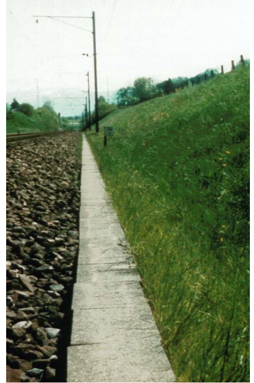
Picture 1 and 2: Concrete border elements (left) and suitably positioned cable troughs (right)
