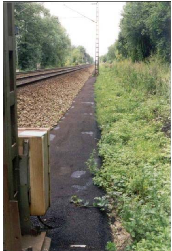
Picture 7 and 8: basalt-granit (left) and macadam thickness 10cm (right)
