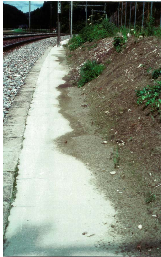
Picture 11 and 12: porous concrete barrier (left), optimised surface (right)
