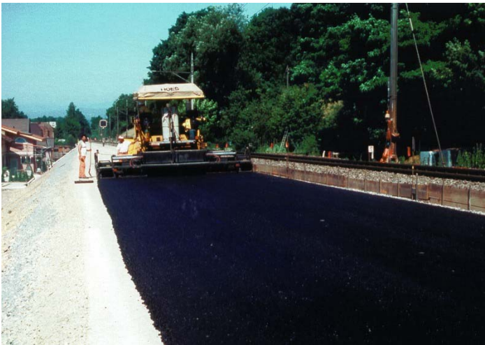
Picture 14 and 15: bituminous layer under the ballast
