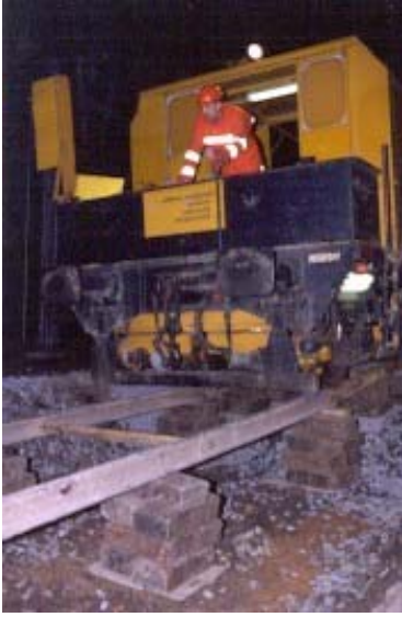
Picture 26, 27 and 28: replacement of ballast with PUSCAL (left), ballast cleaning (right)
