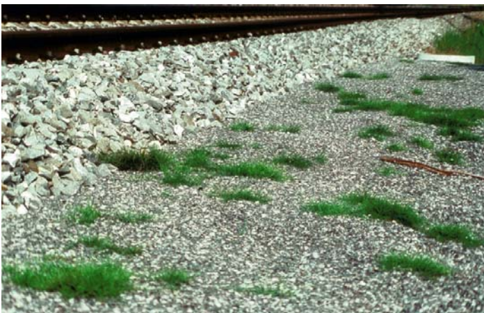
Picture 18 and 19: use of penetrable foils: penetrated by horse-tail
