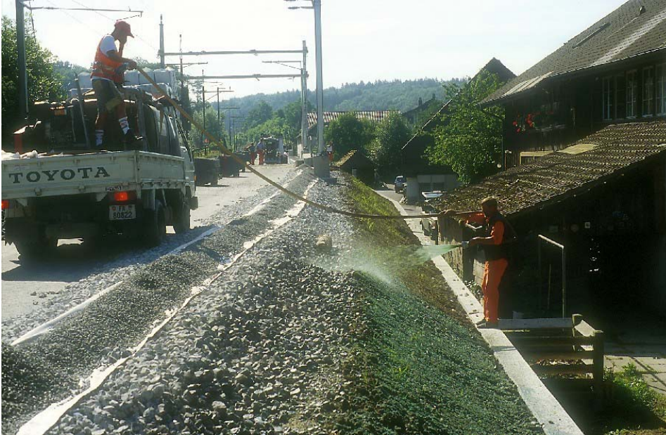
Picture 21: Greening with non ingrowing plants right after construction
