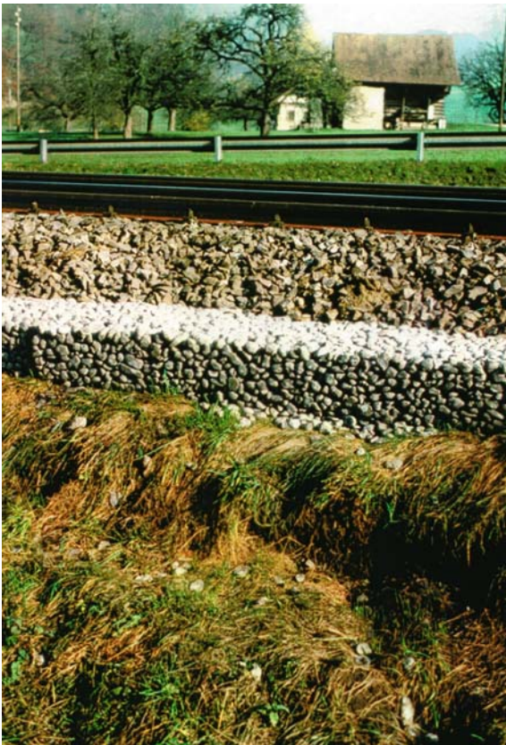
Picture 11 and 12: porous concrete barrier (left), optimised surface (right)
