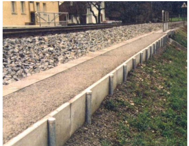
Picture 1 and 2: Concrete border elements (left) and suitably positioned cable troughs (right)
